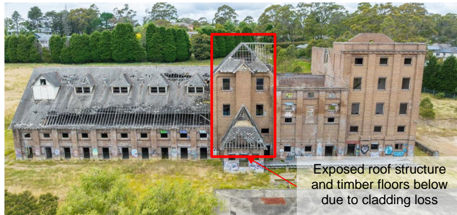
Figure 4: M3 kiln room timber roof condition
