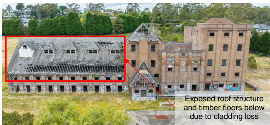
Figure 3: M3 machinery room timber roof condition
