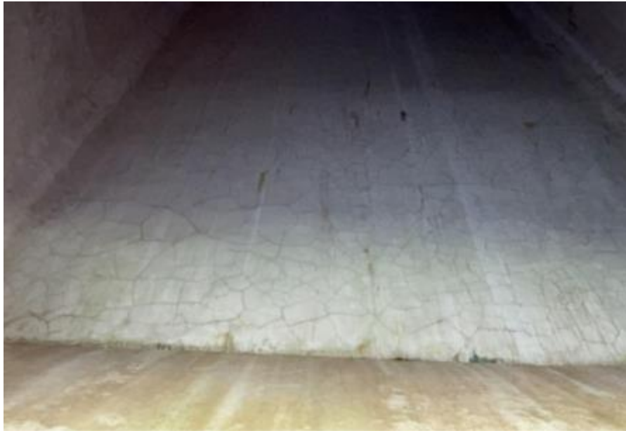
Figure 5: Map cracking on M3 silo internal topping
